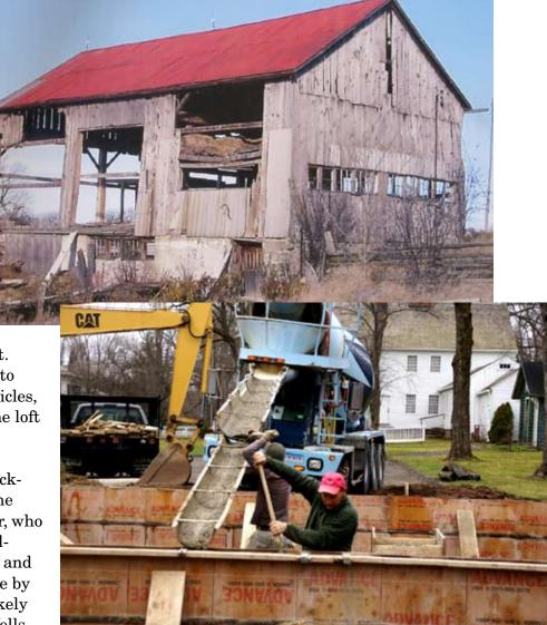
Top: The Society's "new" old barn, shown here before it was fully disassembled in Canada, is being erected at the King House Museum. Lower: As concrete is poured for the new barn foundation, Doug Colson spreads the mix along the form as Brandon Stafford encourages the flow from the trough.
